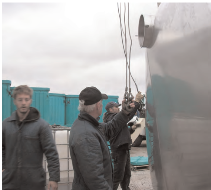
John Neufeld Jr and John Neufeld Sr inspect one of the six new stainless steel tanks upon arrival at the winery. Our capacity is now up another 540,000 litres.
